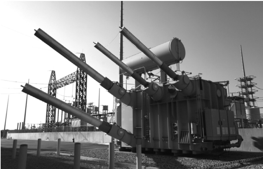
Spare Transformer at Duffy Street Station, Neptune Project
